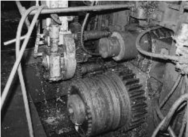
SO/SX Sprag Clutch used as an overrunning device on a nip roll in a steelwork rolling mill. Speed overrun is often created by the steel being rolled.
